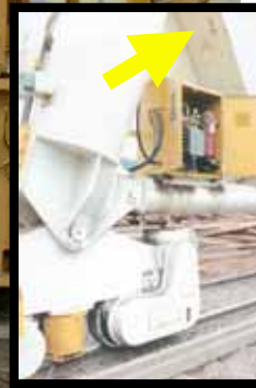
Guard over control box
